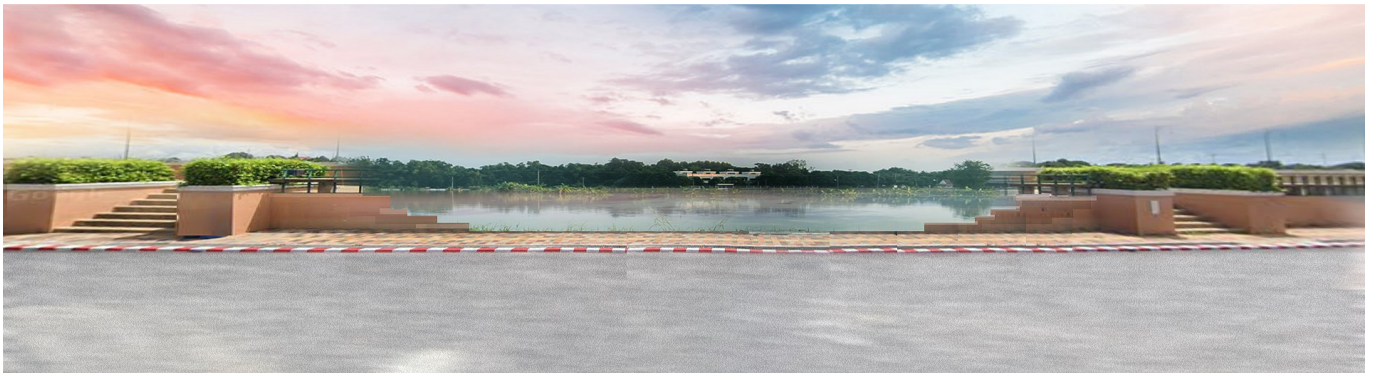
A conceptual image of the Self-Closing Flood Barrier system during normal water levels. The flood barrier is concealed underground, keeping the riverbank area open, easily accessible, and unobstructed, preserving the view.
